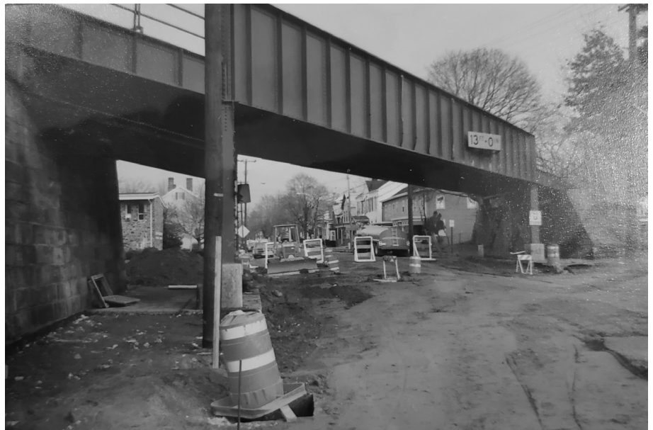
Removal of the C&A train trestle over Main Street
